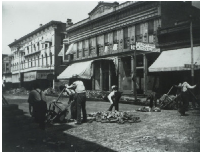
Workers installing brick pavers along South Randolph Street in the late 1800s [Western Illinois University Archives & Special Collections]
