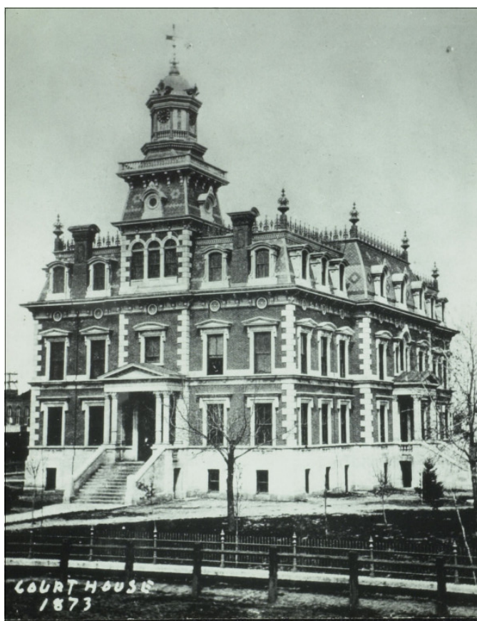
The courthouse building soon after completion. Note the original mansard roof, which was converted to a side-gable roof in the late 19th century. [Western Illinois University Archives & Special Collections]
