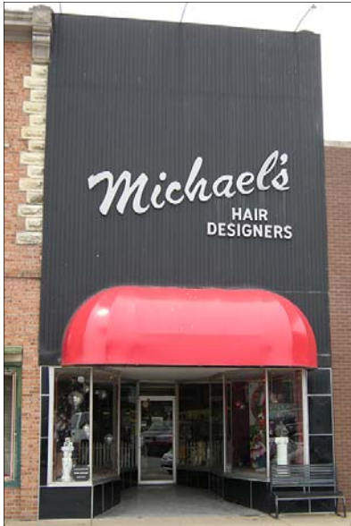
Metal sheath covering façade of 22 West Side Square
