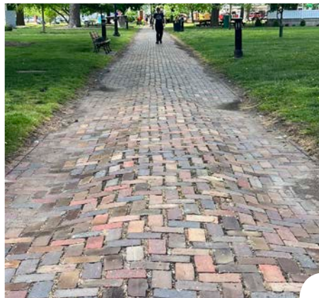
Brick paver walkways, uneven and rutted from vehicular use
